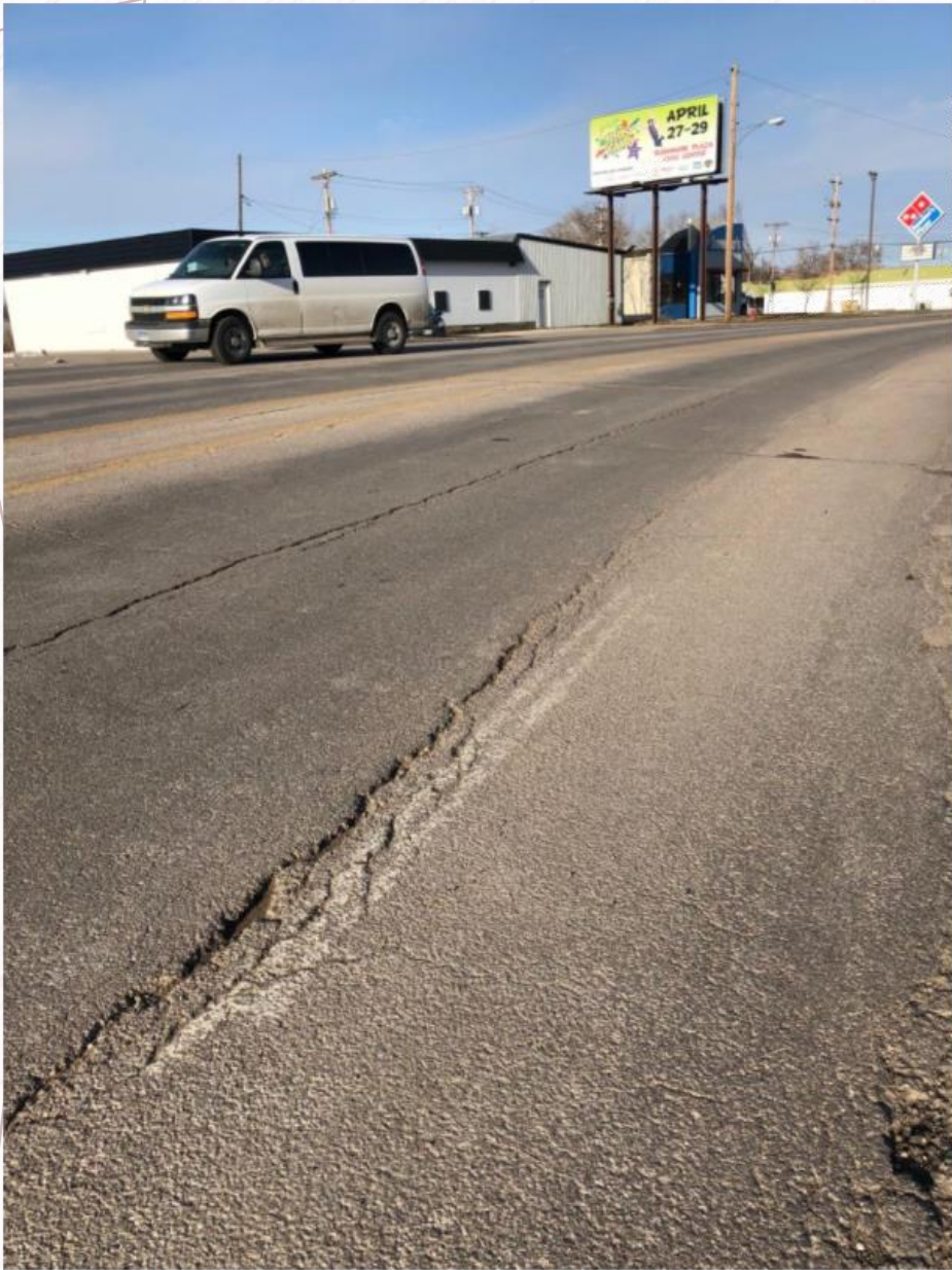
Even on a sunny day, the white lines are almost invisible between the lanes on this busy, curving section of East North Street in Rapid City. City officials say they repaint the lines each year, but tire wear, weather and plows wear the markings down each winter. Photo: Bart Pfankuch
